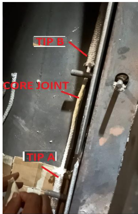
Figure 10: Core joint making points using masking
