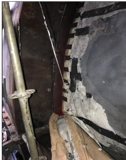
Figure.13. (a) Insulation arrangement (refer MLI 0816)
